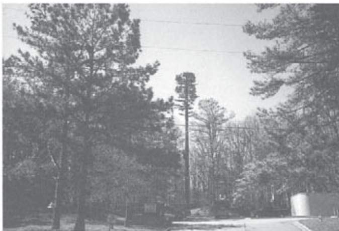
Fig. 9. Cellular antenna tower disguised as a tree.
